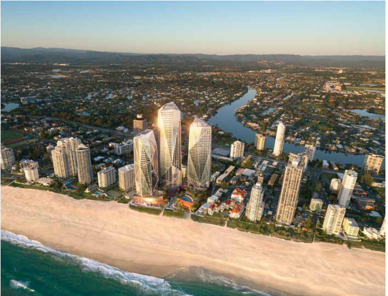
The three towers of the Jewel complex – the tallest of which is 170m – rise above Australia's Gold Coast
