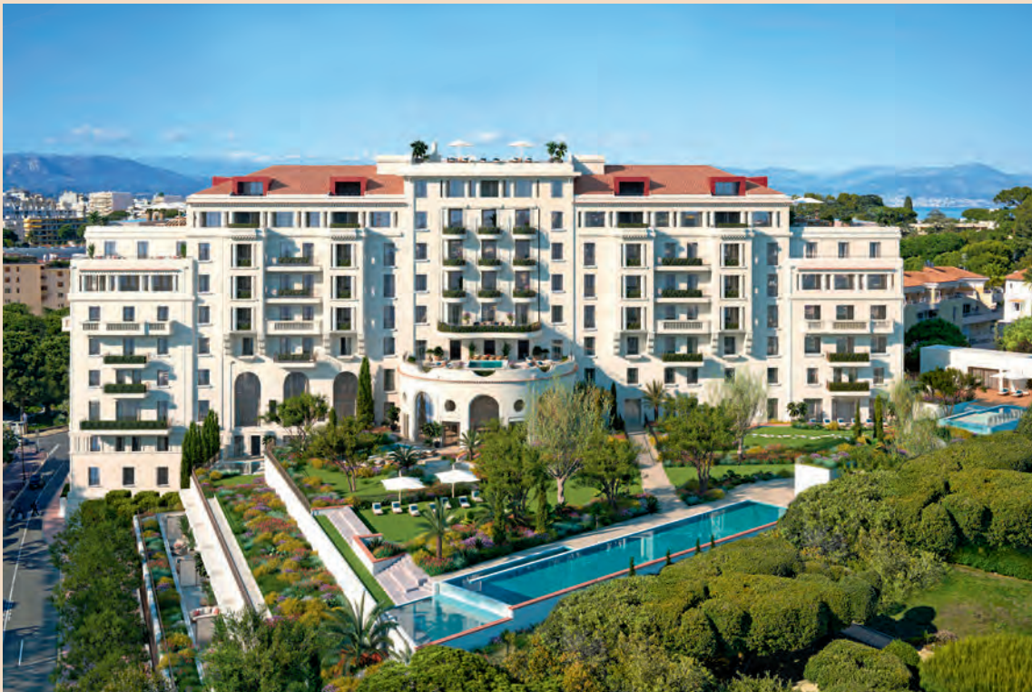
The magnificent façade of Cap d'Antibes' 39-residence Le Provençal complex
